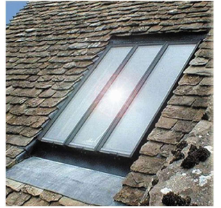
ROOF LIGHTS Conservation style rooflight "the rooflight company" or similar. To be flush with flat roof and hidden by parapet.
