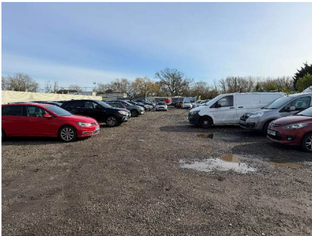
Photograph 5: View of main yard car storage area showing road planings surfacing, facing east.
