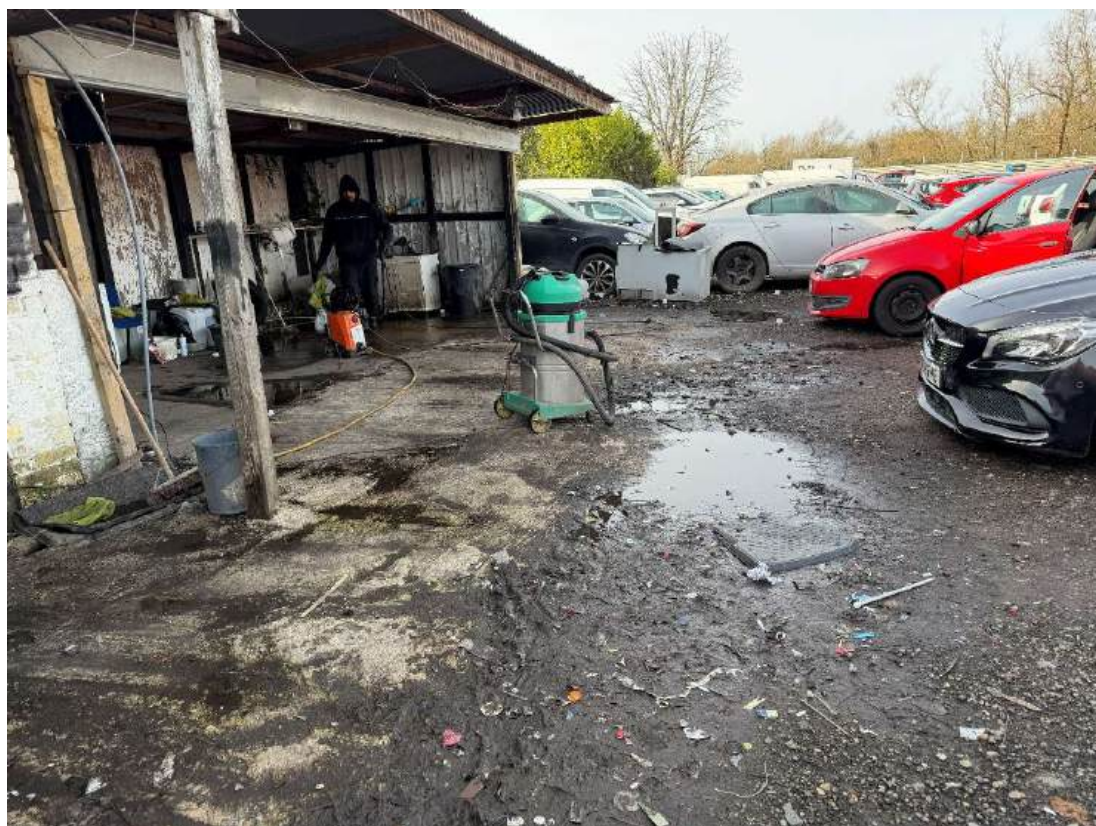
Photograph 4: View of structure along southern boundary, currently used as a car wash facility, facing west.
