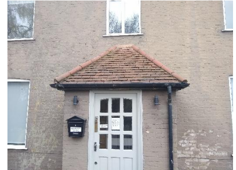
Porch structure to frontage
