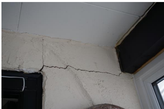
Front Elevation - Horizontal crack to right of front door
