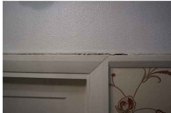
Hall - Drop in lounge door frame
