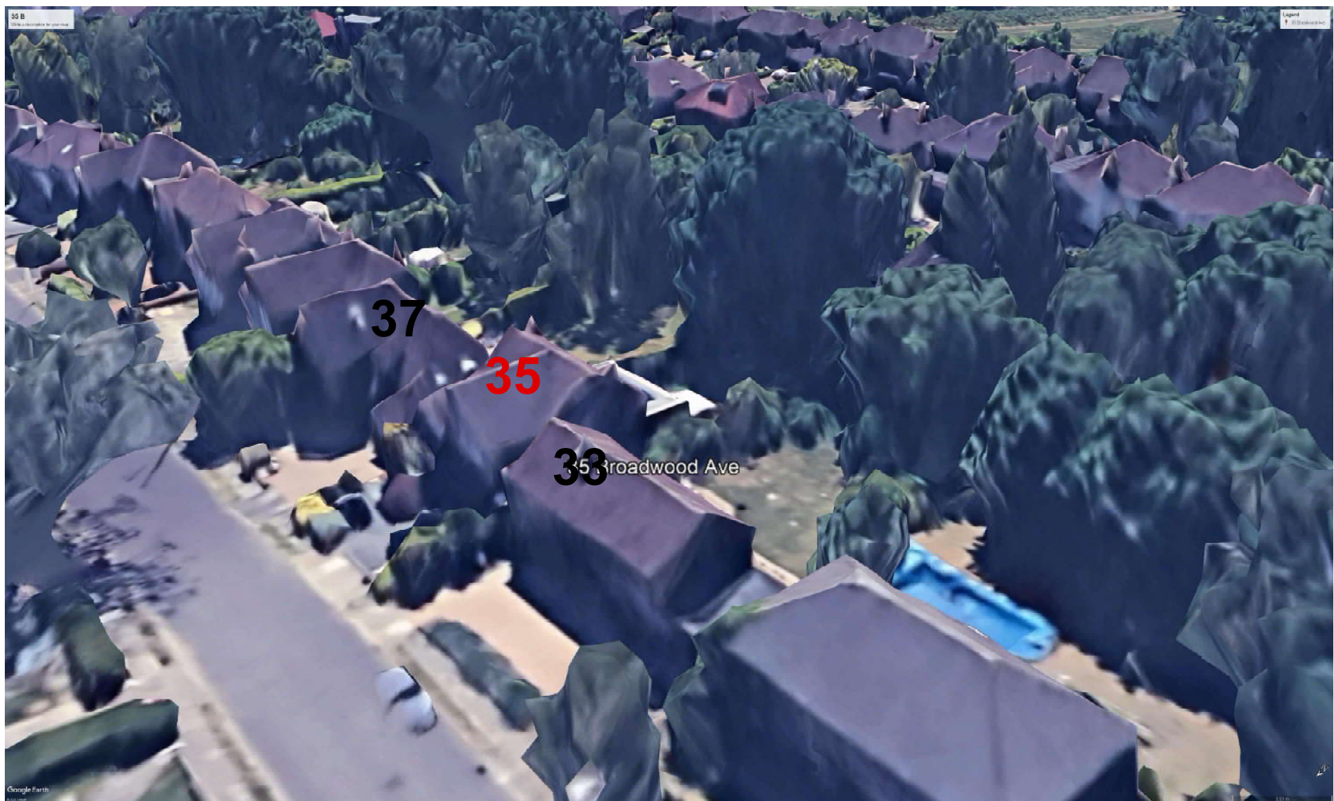
AERIAL VIEW showing application property 35 Broadwood and neighbouring properties 37 Broadwood and 33 Broadwood
