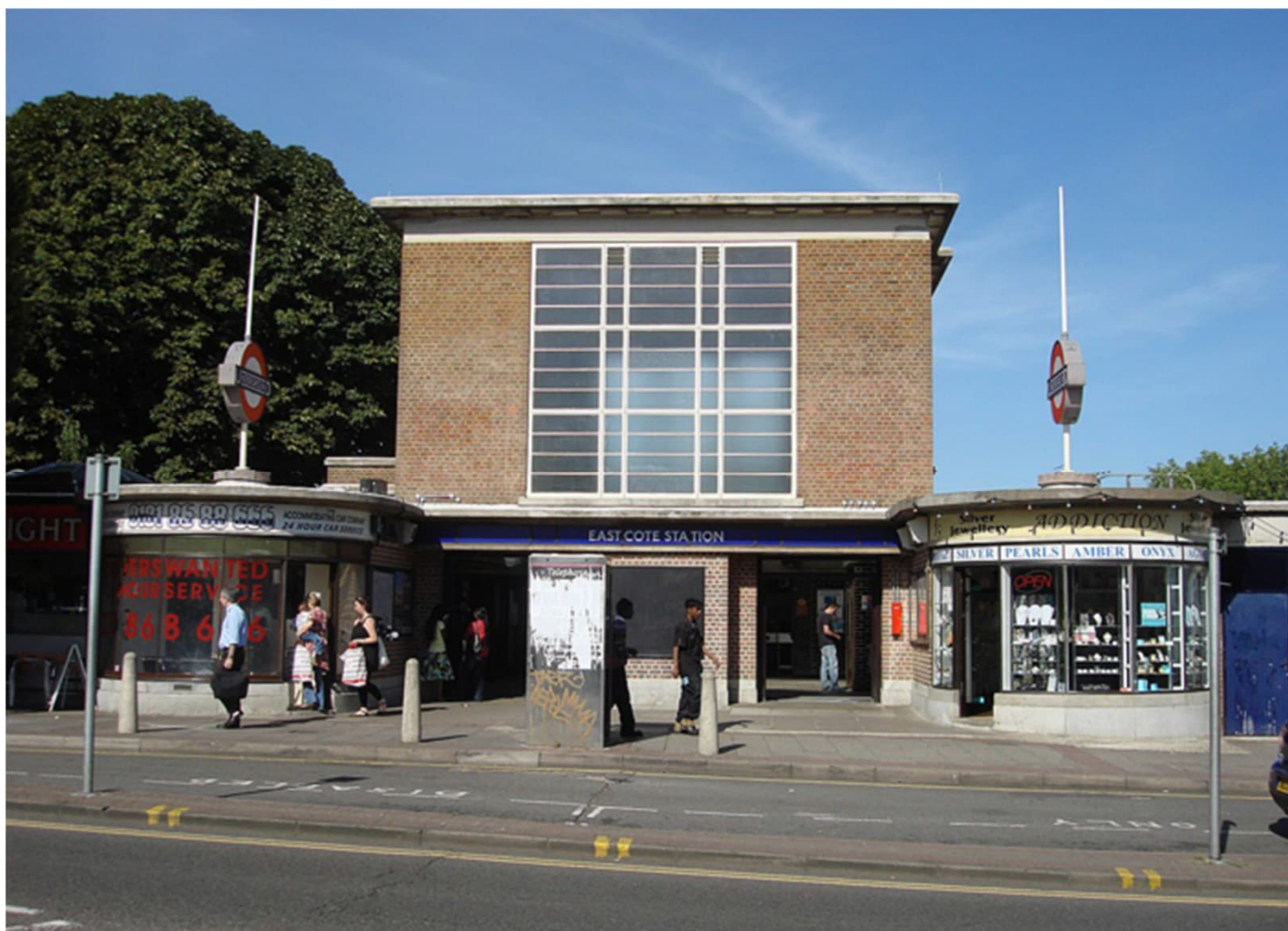
Eastcote Station - Existing Station Entrance
