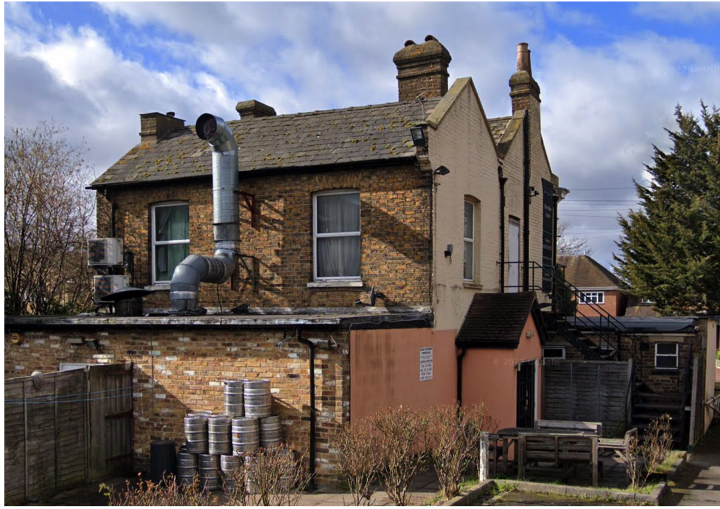
Rear of Existing Former Puclic House
