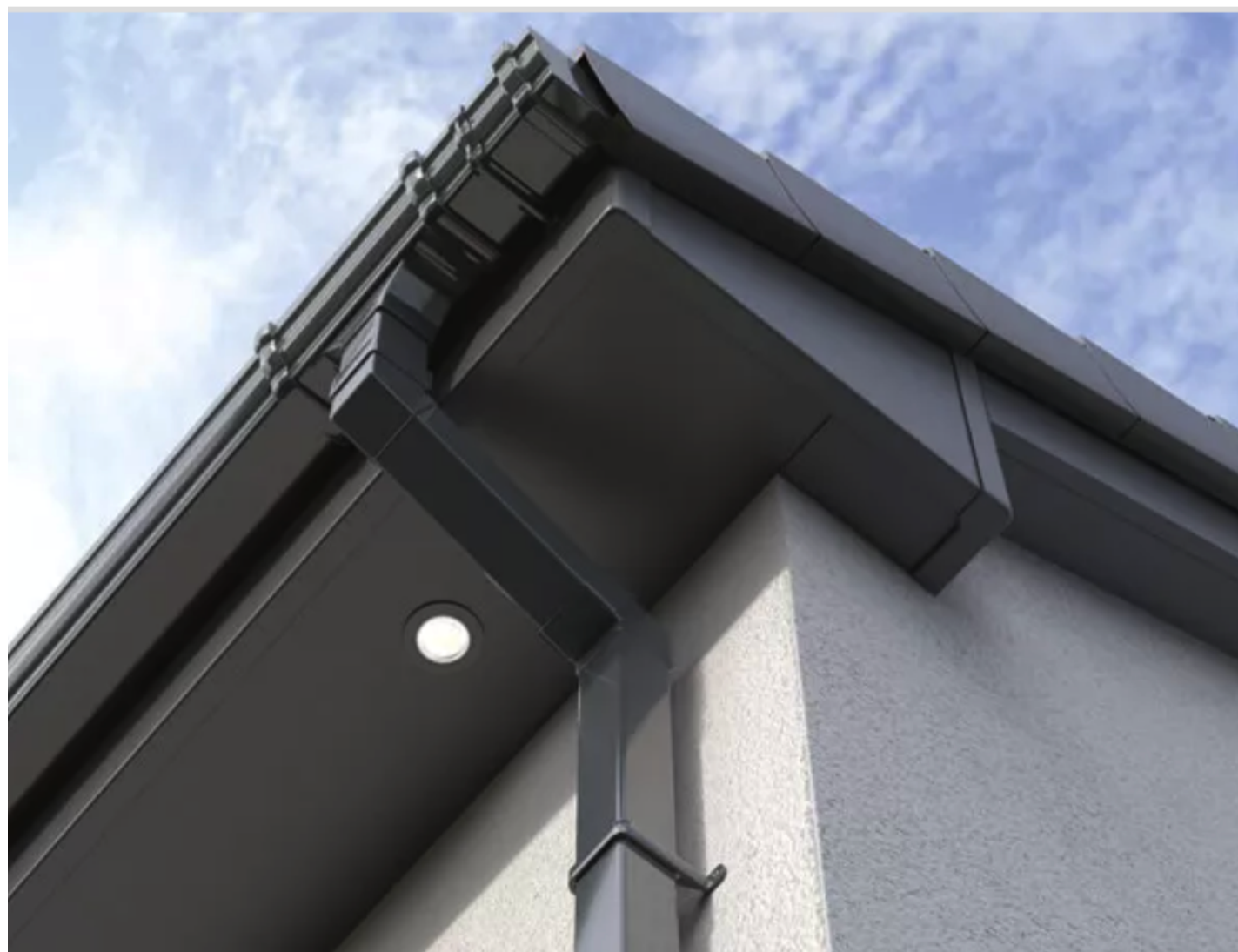
2 Grey uPVC Rainwater Goods and Soffits
