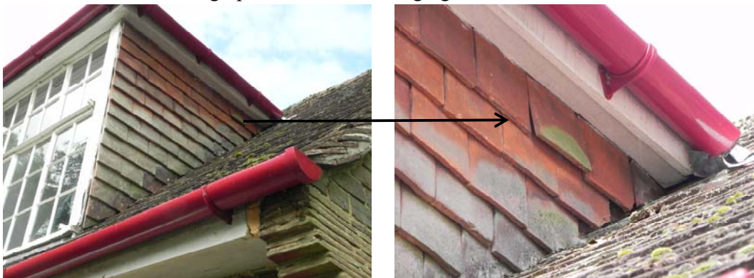
Photograph 12-13: raised hanging tile rear dormer
