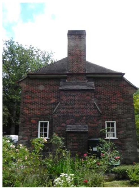
Photograph 11: side (southwest) elevation
