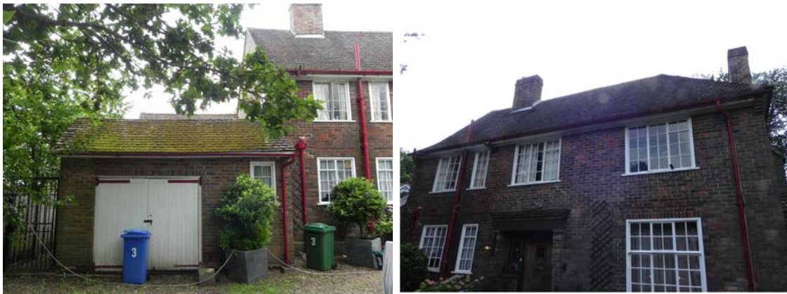
Photograph 6-7: front (northwest) elevation
