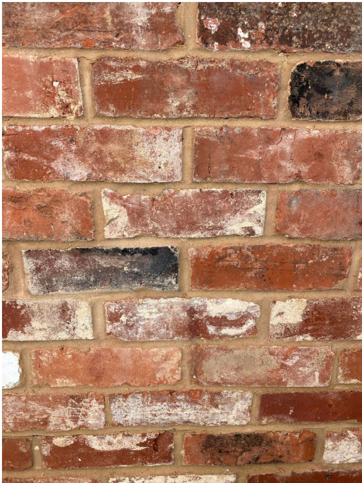
Wire cut multi brick slips manufactured on site from same batch as already used in all elevations
