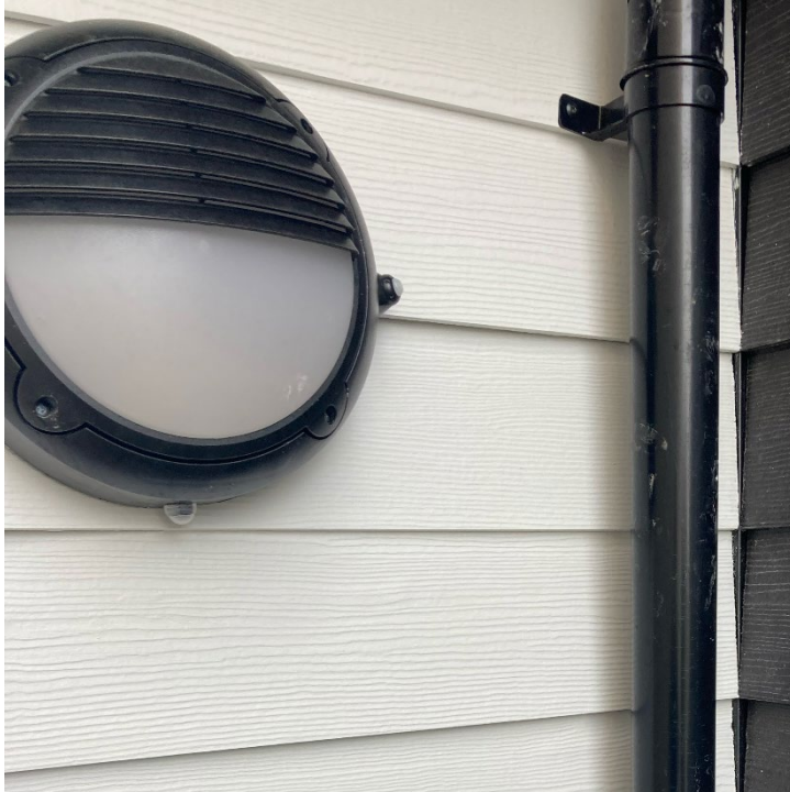
Zinsser RAL 9016 exterior grade satin paint finish applied over original finish
