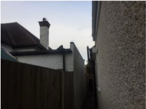
Side access between no. 7 and 9
