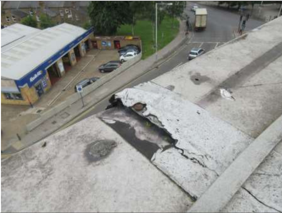
03: Defective pressed coping joint
