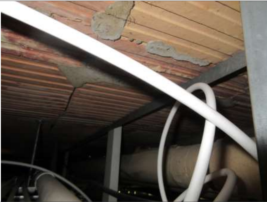
05: Screed hollow pot clay floor at 1 st – 3 rd floor levels
