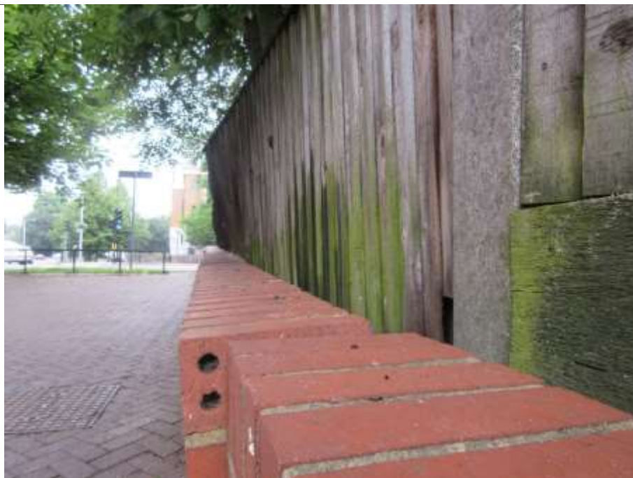
14: Section of north boundary wall and block paving suffering from ground heave
