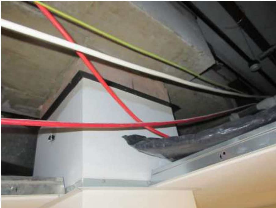
04: Concrete column junction with concrete roof slab
