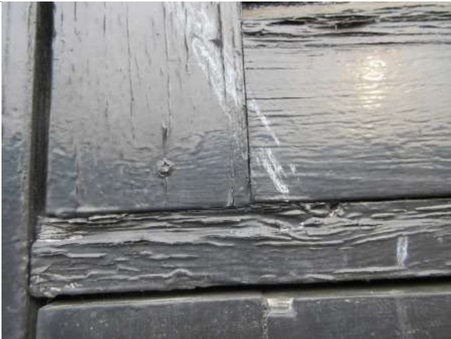
10: Defective paint finishes to external timber features
