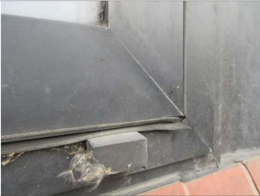
09: Loose seal to openable window
