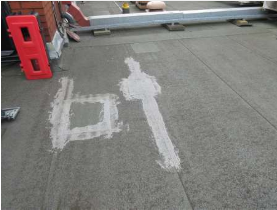
01: Historic repairs to roof covering
