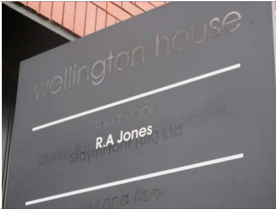
13: Significantly solar faded totem signage to main entrance
