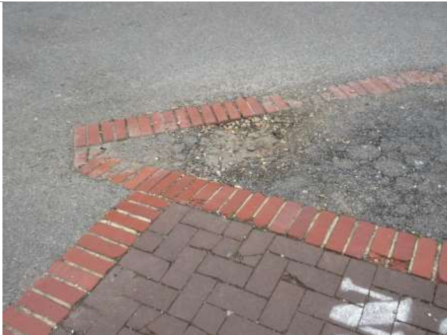
12: Damaged and uneven macadam surfaces and blockwork demarcation to rear car park
