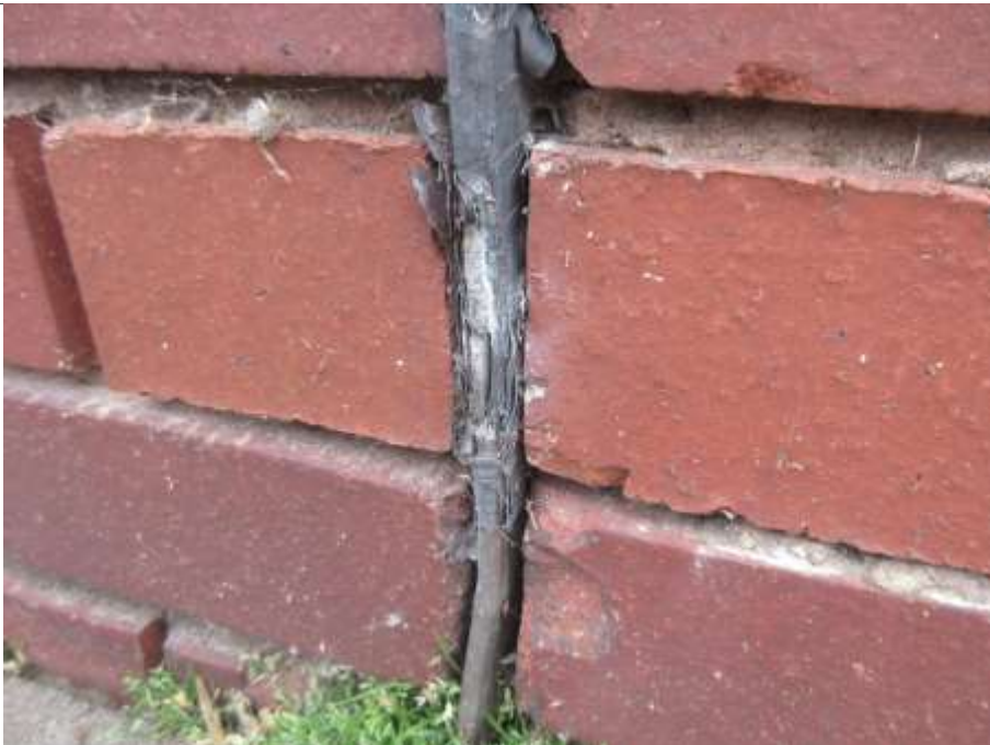
08: Degraded mastic infill to East elevation expansion joint
