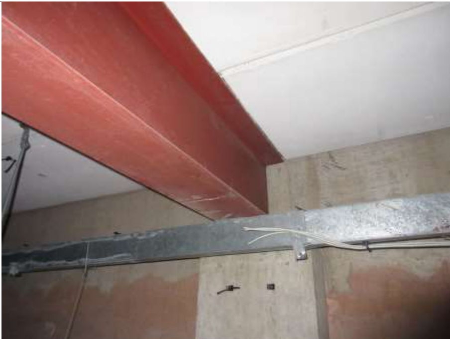
06: Pre-cast concrete planks overlaying steel I-beam roof raft member
