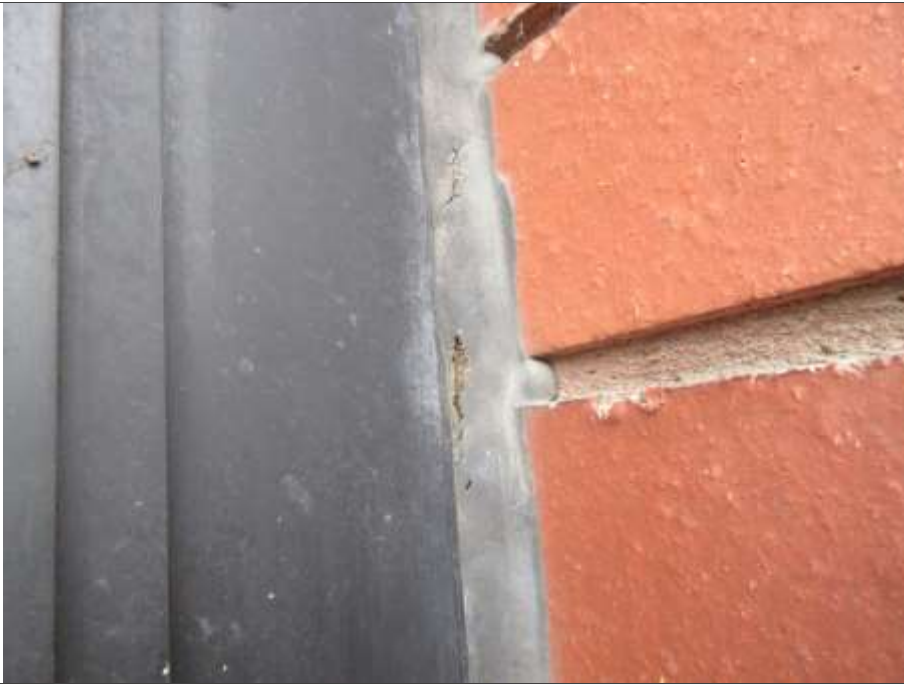
07: Degraded mastic seal to window reveal
