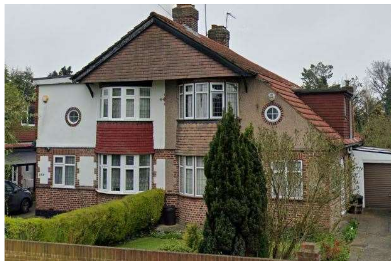
Front elevation of nearby 270/272 Long Lane using brick detailing to subdivide light and dark rendered elements
