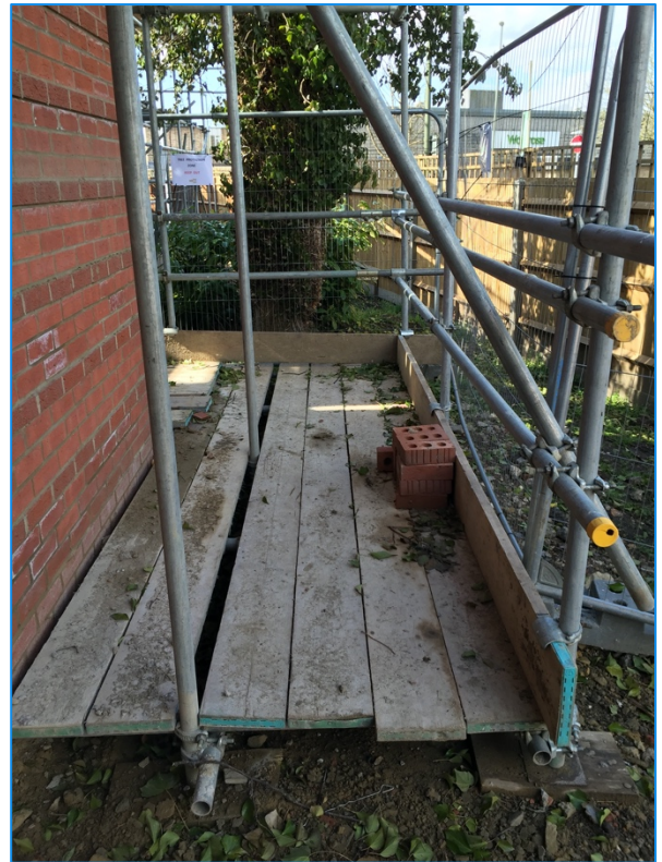
Scaffold ground protection
