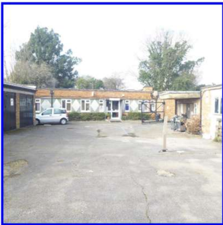
Rear Yard & Unit 4
