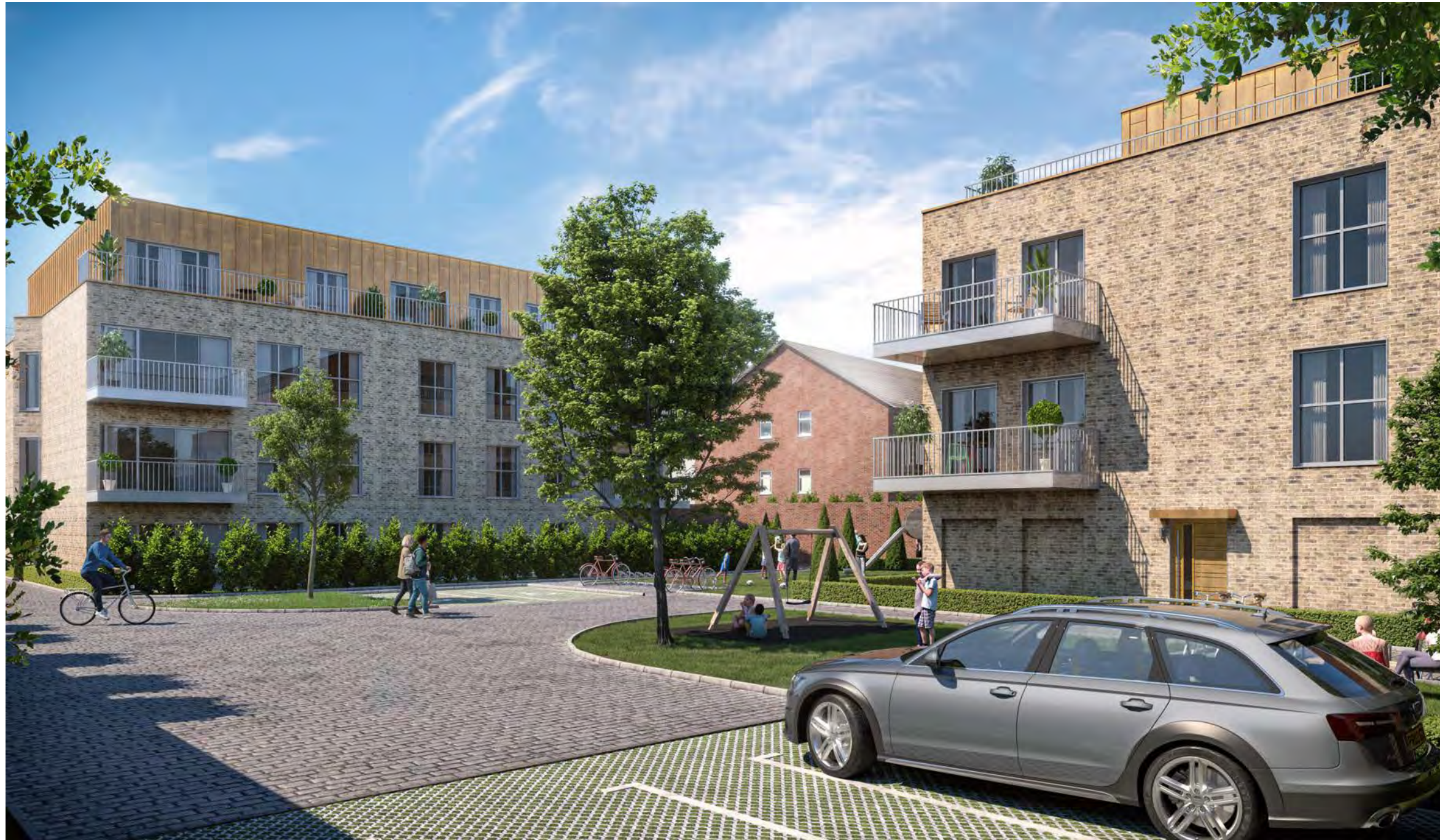
View towards block 1 from central area of site
