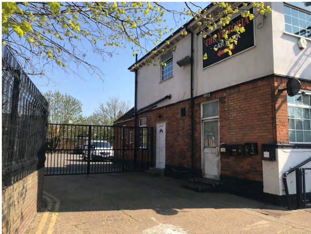
1 View of west side of Victoria Pub
