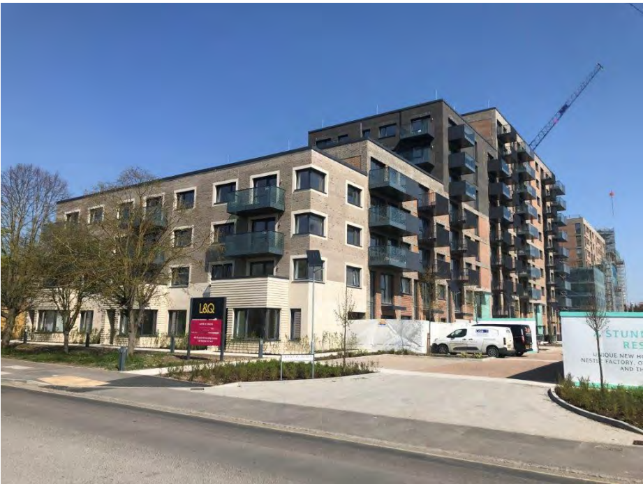
Hayes Village residential block under construction on the former Nestles site (Site A)
