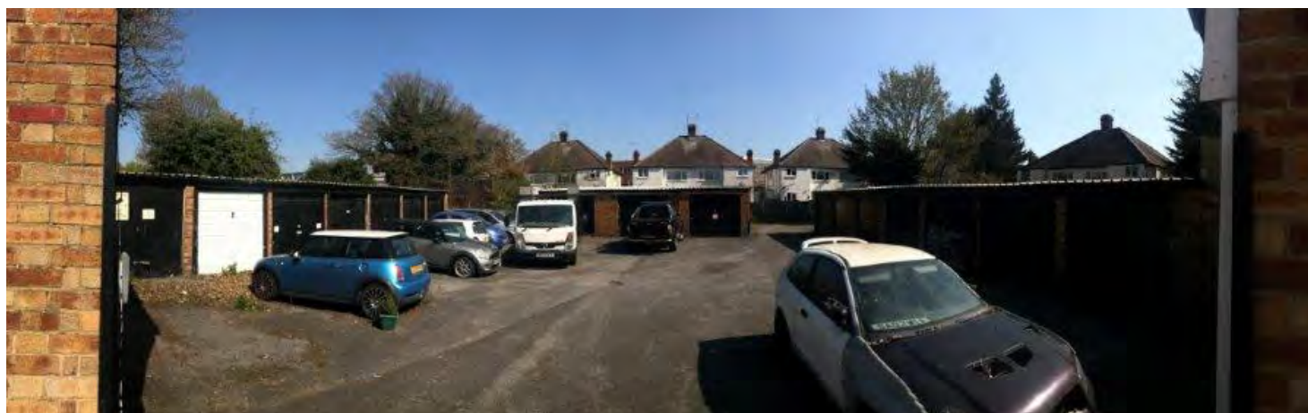
2 View into garages site
