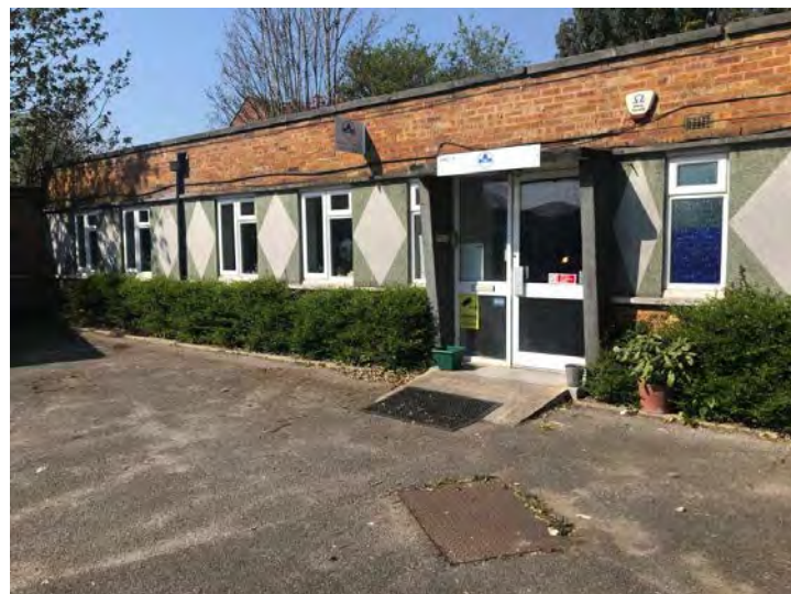
3 Offices in garage site
