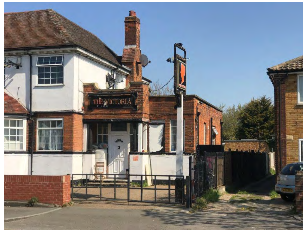
1 View of east side of Victoria Pub
