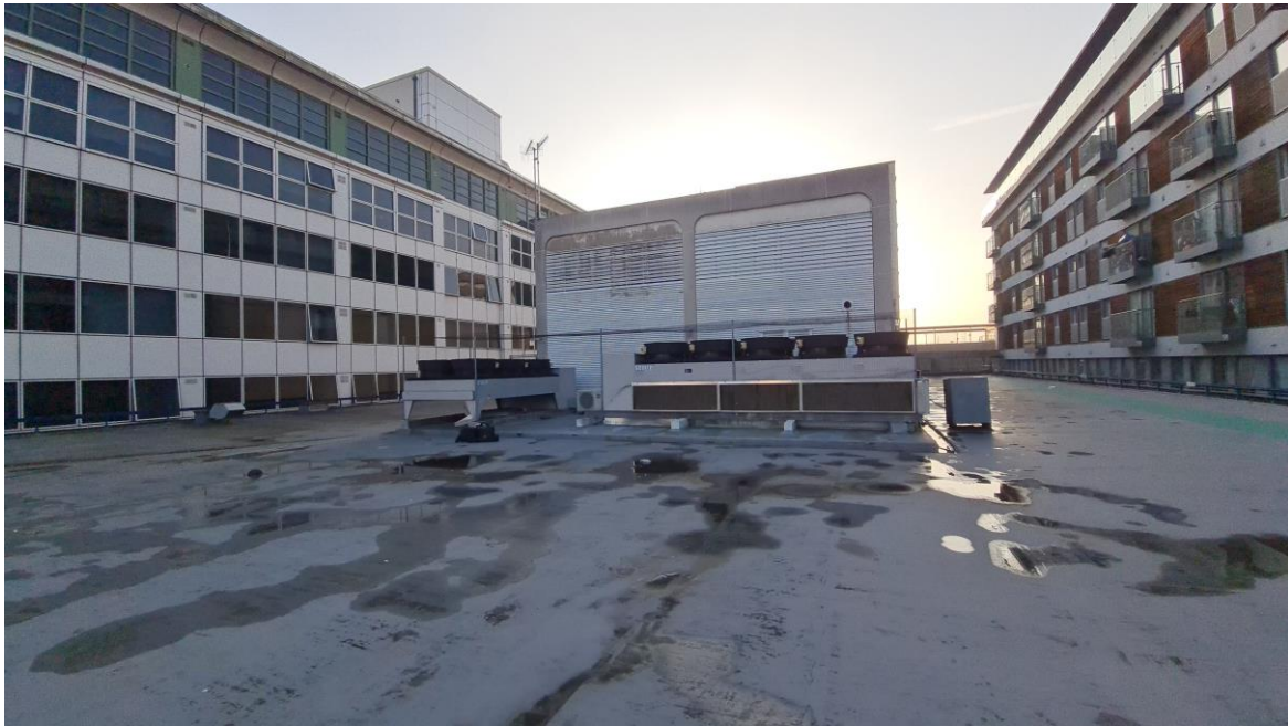
FIGURE 3: Current refrigeration condenser units to be replaced.
