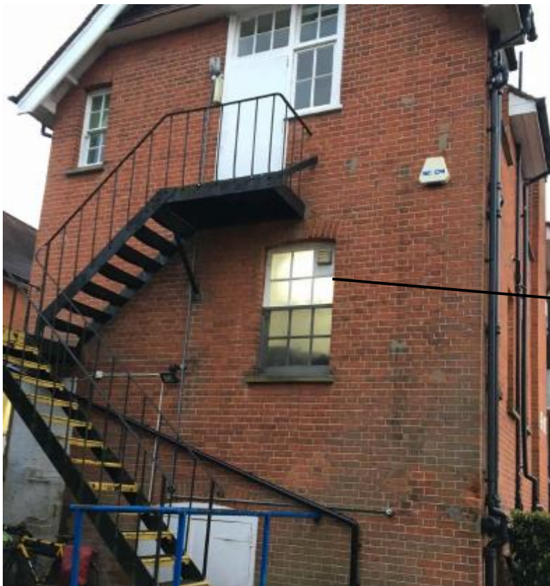
Photo of the western elevation of the catering block
