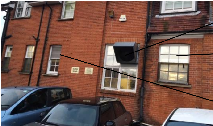
Photo of the southern elevation of the catering block
