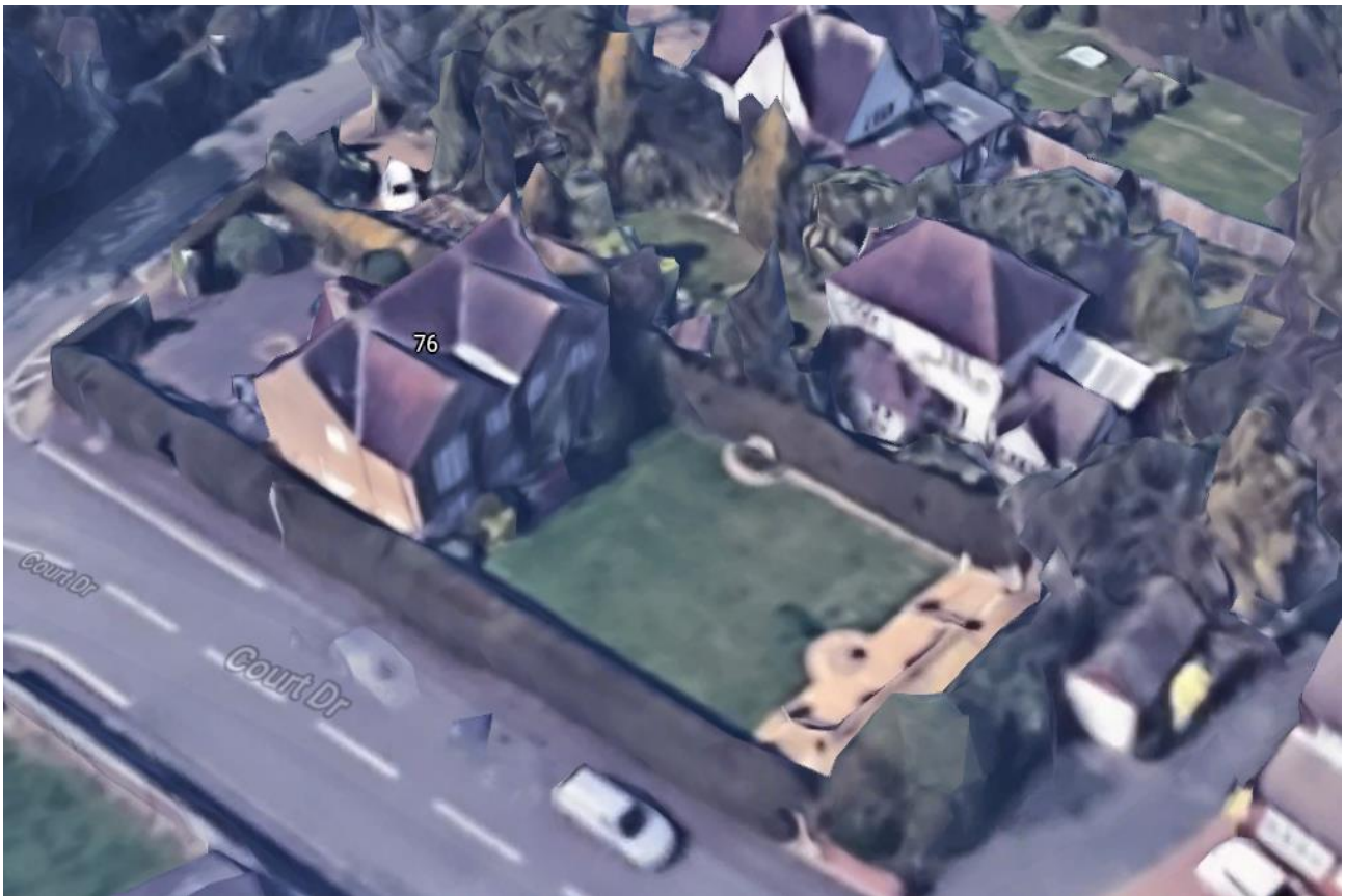
Image 3 - Overhead view of the rear of the site demonstrating the existing relationship between 76 and 78 Vine Lane
