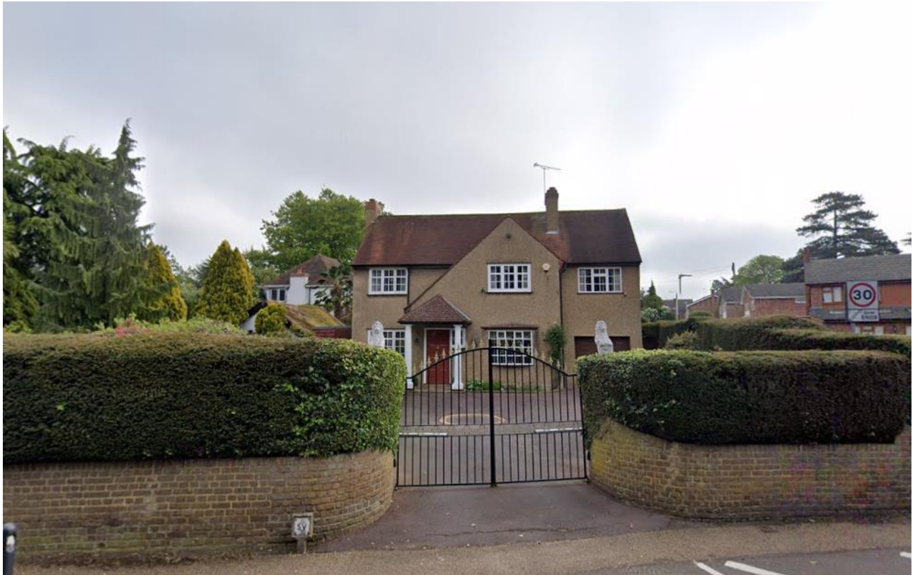
Image 1 – View of front elevation from Vine Lane
