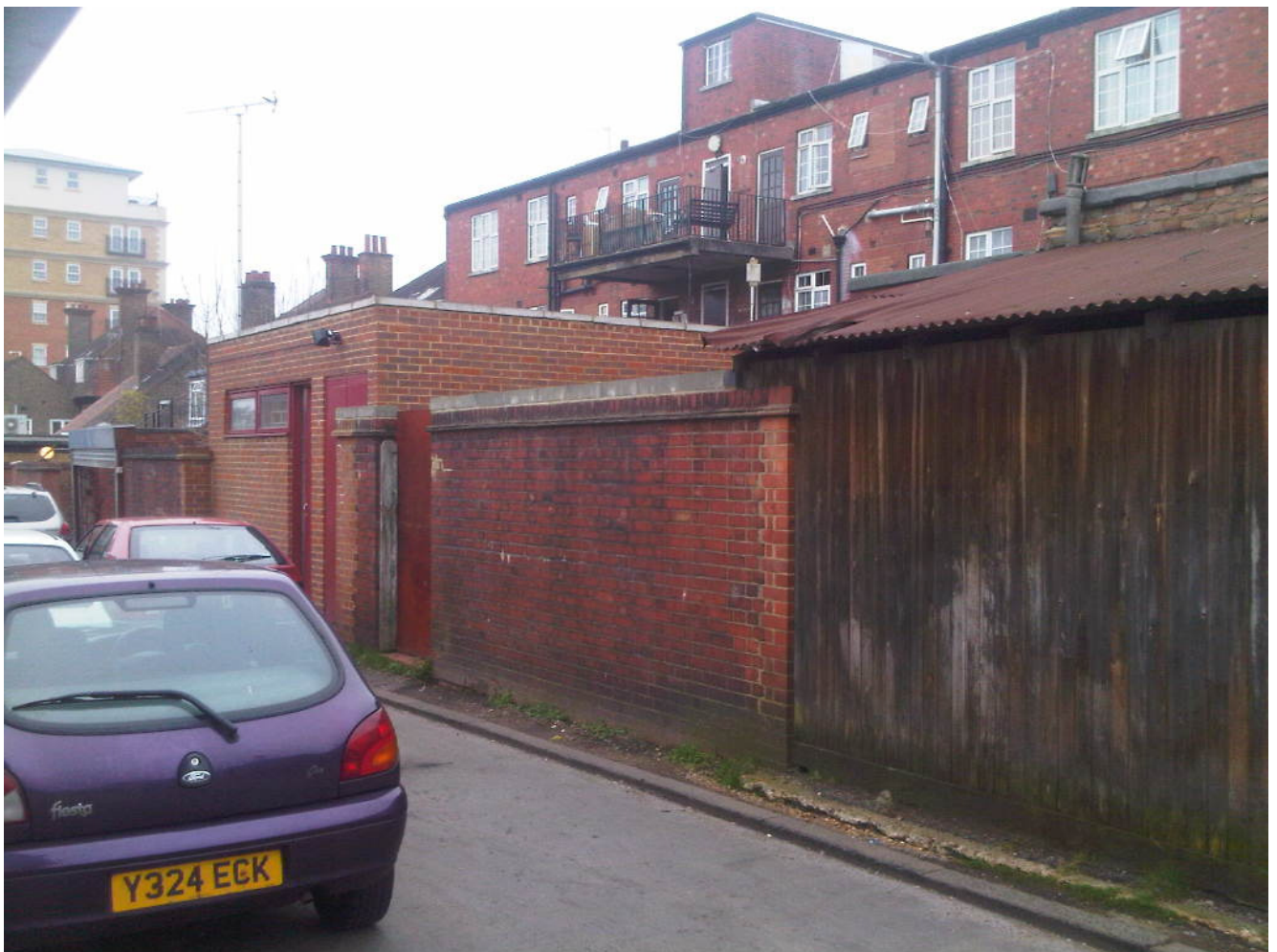
Figure 5 - Rear access to the property
