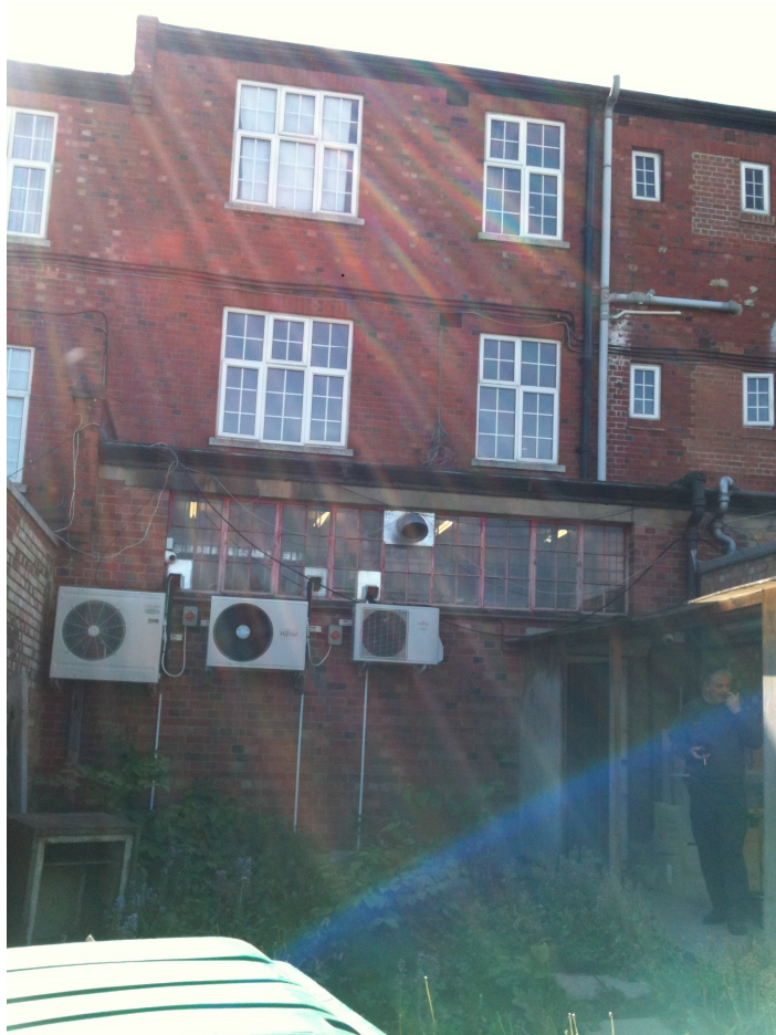
Figure 3 - Rear of 135 High Street
