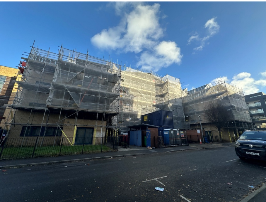
Figure 2. Union Wharf - Front elevation - Remediation works
