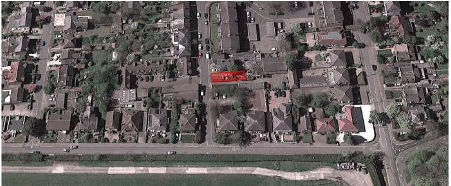
Aerial View Looking West
