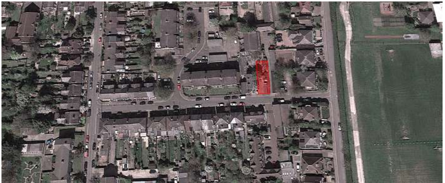
Aerial View Looking North
