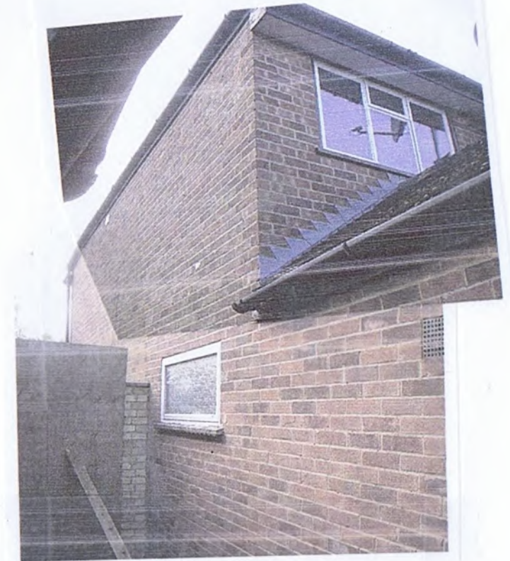
side of No 58, viewed from the side passageway.
