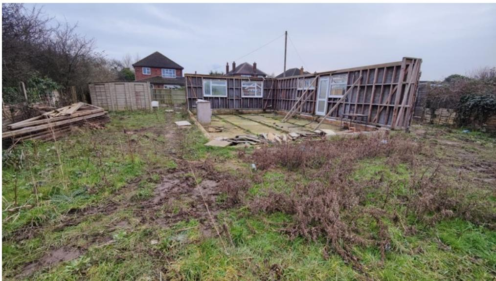
2. It is estimated that there is about 20-40KG of Asbestos used in the garage roof being demolished. The materials will be carefully ceased and packed by a qualified contractor and will be disposed as per the process stated by Hillingdon council <https://www.hillingdon.gov.uk/article/2342/Disposing-of-asbestos>
