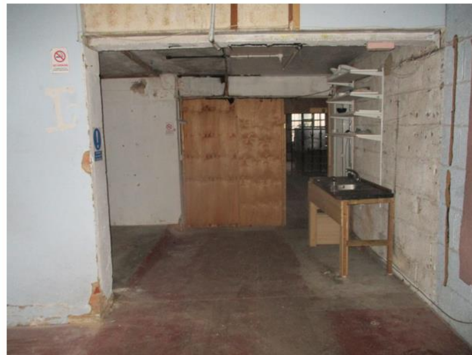
Photo No.16: Facing north from the same spot looking towards the entrance to unit No.18 from unit No.20 (right)
