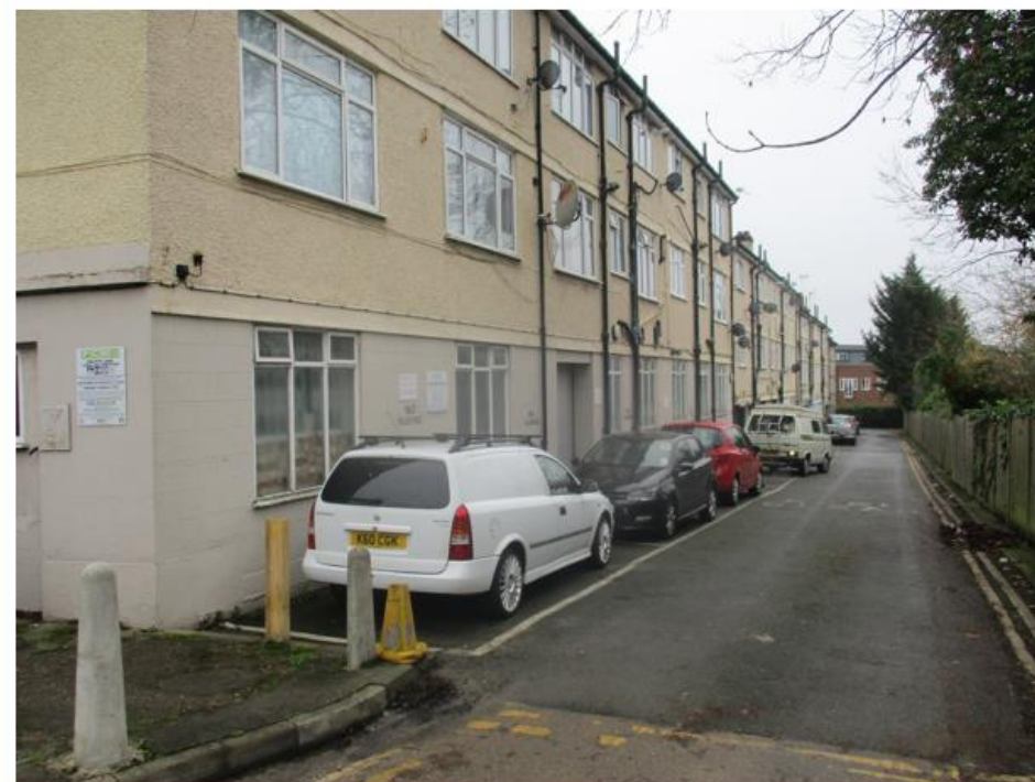
Photo No.2: Facing east from the same location showing the southern face of the building and access road to eastern extent
