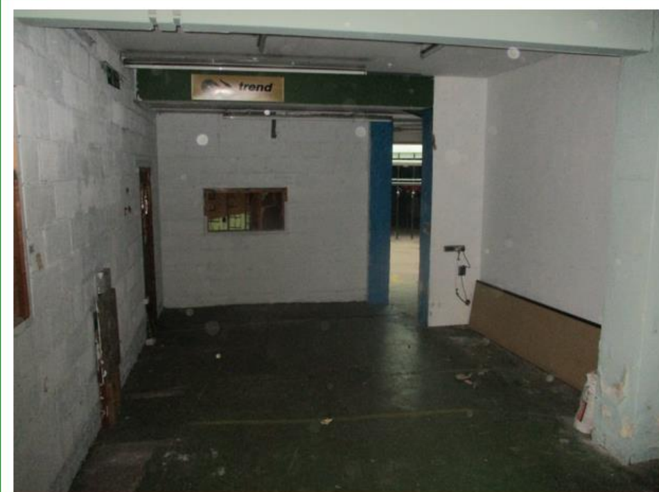
Photo No.8: facing east inside the access to units No.2-6 showing unoccupied, former commercial floorspace
