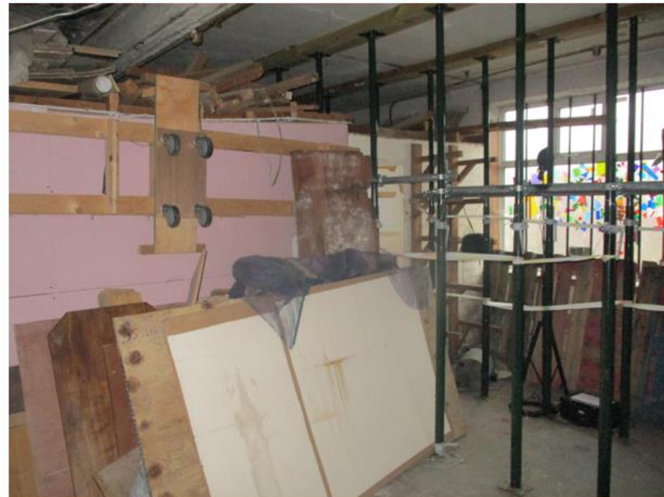
Photo No.20: Facing NW from the same spot showing a toilet enclosure in the far NW of units No.18/19
