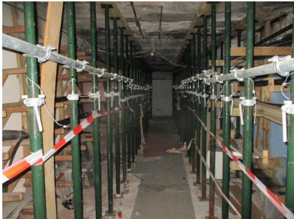
Photo No.19: Facing slightly SE from the NW extent of units no.18/19 showing further supporting acrows and shelving
