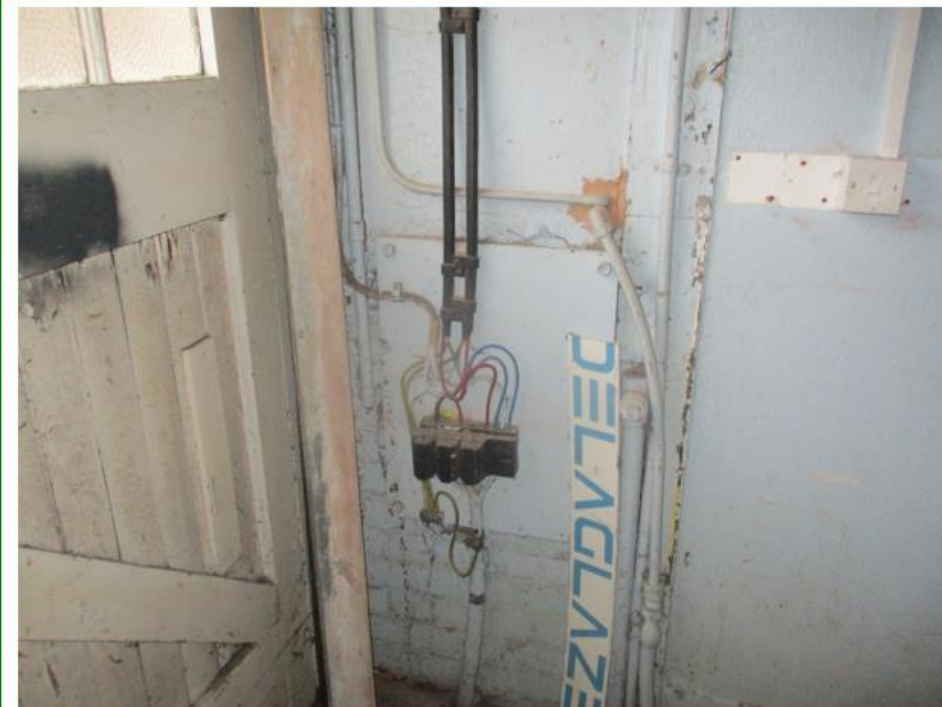
Photo No.30: Service entry noted on the southern face of the building in unit No.22
