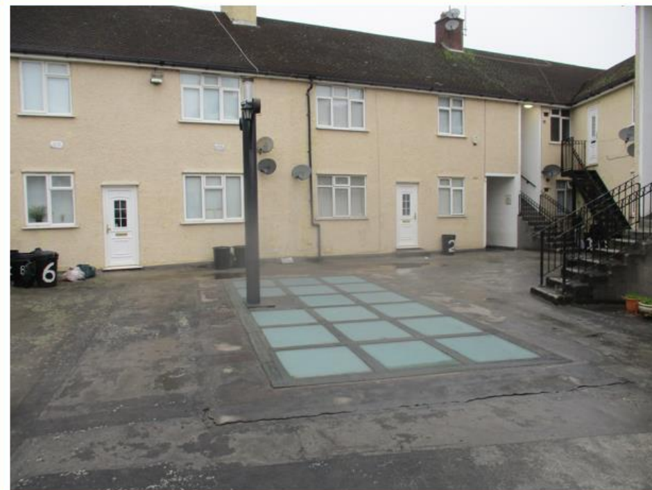
Photo No.6: Skylight and stack of units No.2-6 noted in the NW extent of the inner, first-floor courtyard of the building
