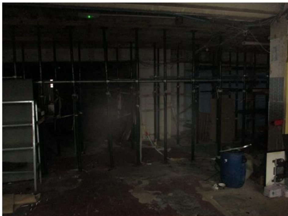
Photo No.17: Facing south from inside the northern face of unit No.18 showing acrows supporting the roofing here
