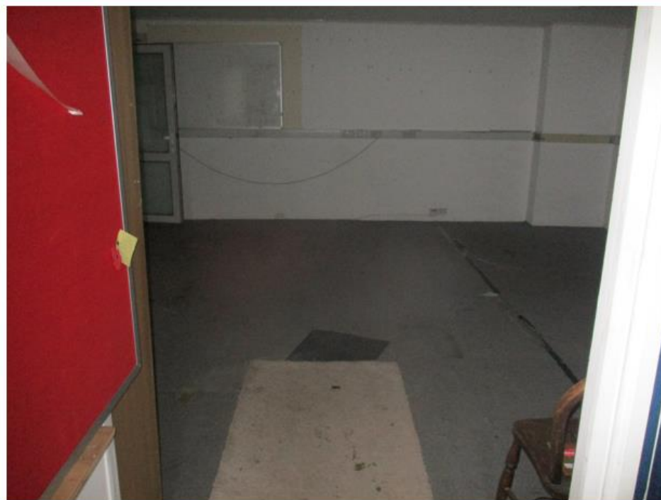
Photo No.14: Facing north from just inside the access of unit No.20 (access to units No.18/19 off to left of photo)
