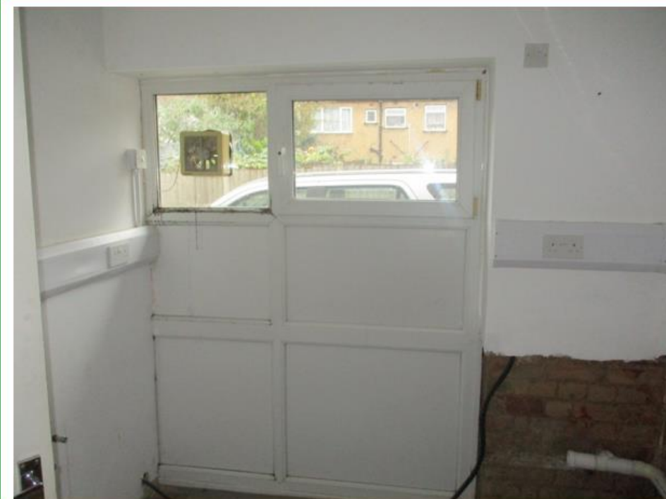
Photo No.24: Facing south from inside unit No.22 showing former office/reception space and service entries
