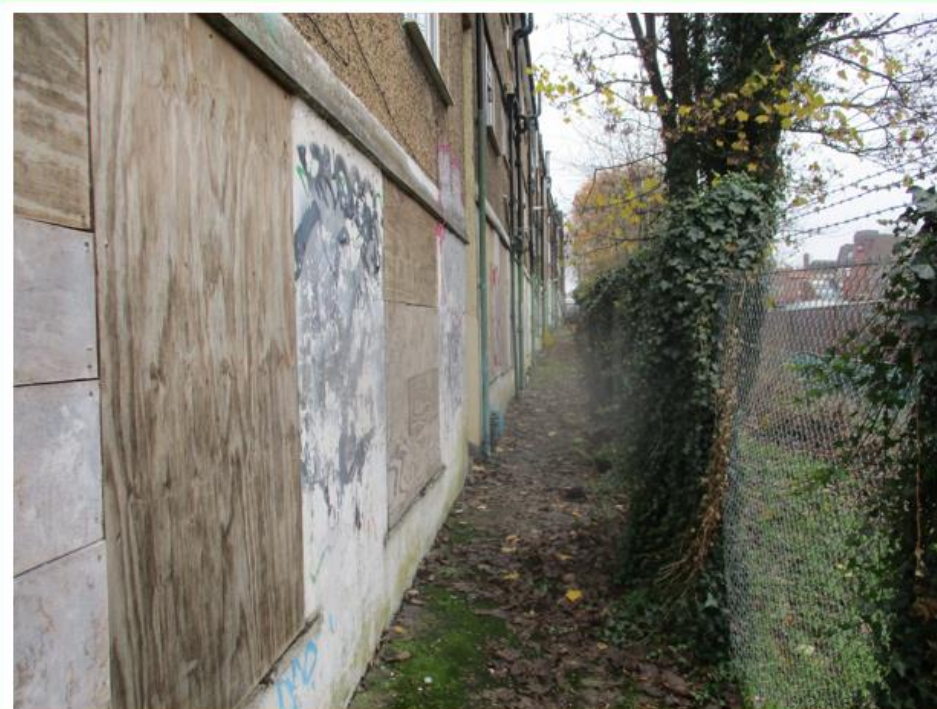
Photo No.4: Facing NW from the NE corner of site showing the northern face of the building and adj. railway (right)
