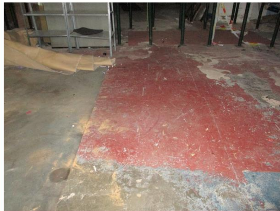
Photo No.18: Example shot of flooring conditions within units No.18-20
