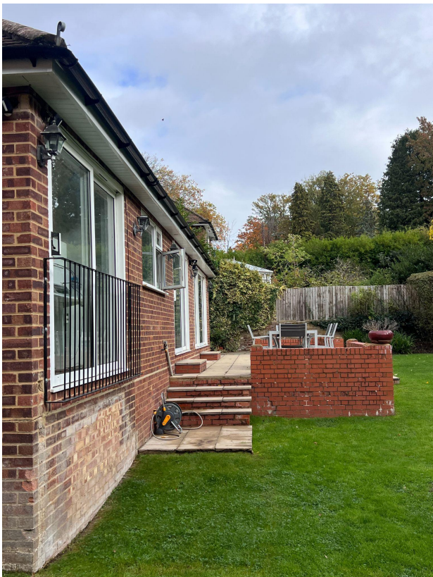
Photo 7 & 8 - Raised rear patio with steps
