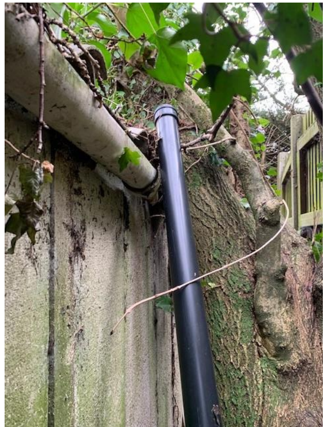
Tree pushing the garage wall/roof
