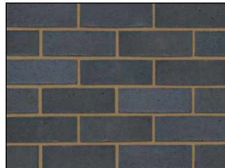
Blue engineering brick - band below DPC
