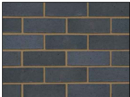
Blue engineering brick - band below DPC
