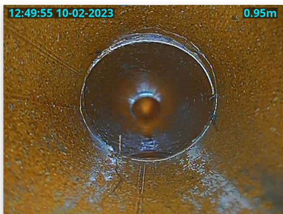
Fig 2.3: Line 3 Cracking
