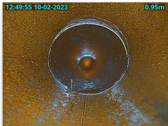
Fig 2.3: Line 3 Cracking
