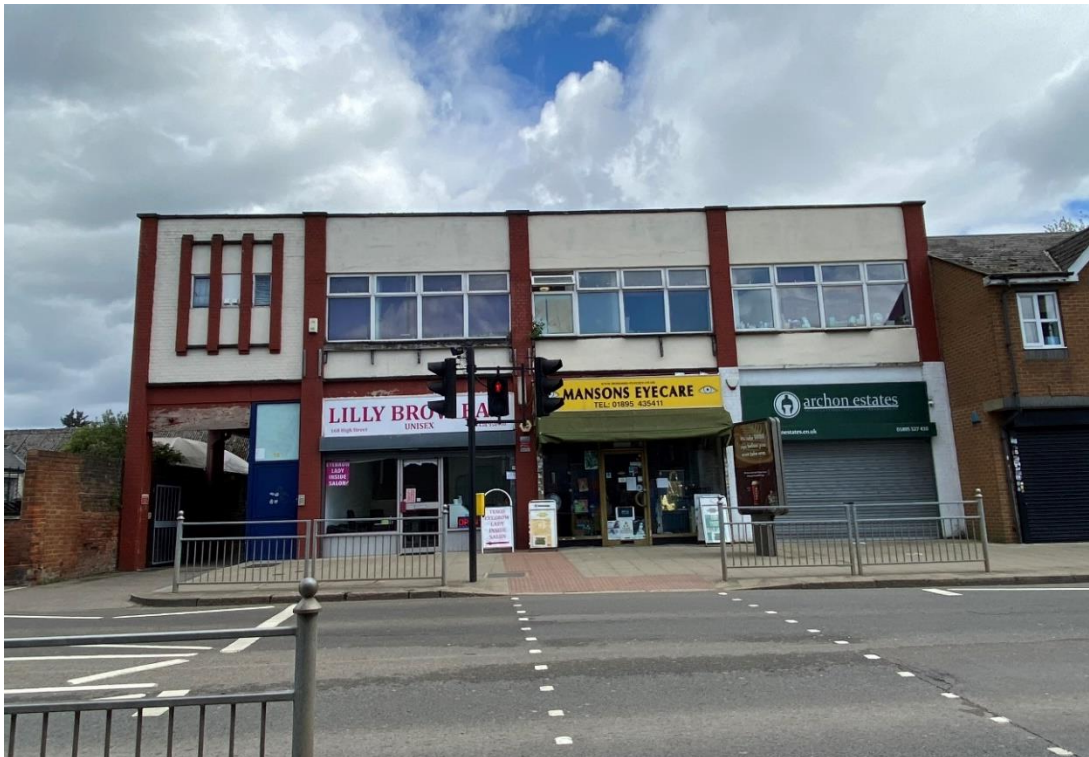
Image 1-Front view of the site with a discordant fenestration, unattractive shop signage and weathered render
