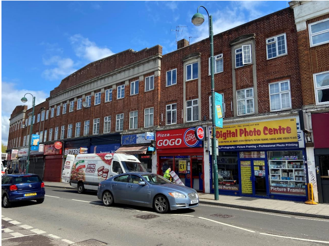
Image 4- Nos 112-134 High Street a three storey terrace with residential accommodation at upper floor levels within Yiewsley District Centre
