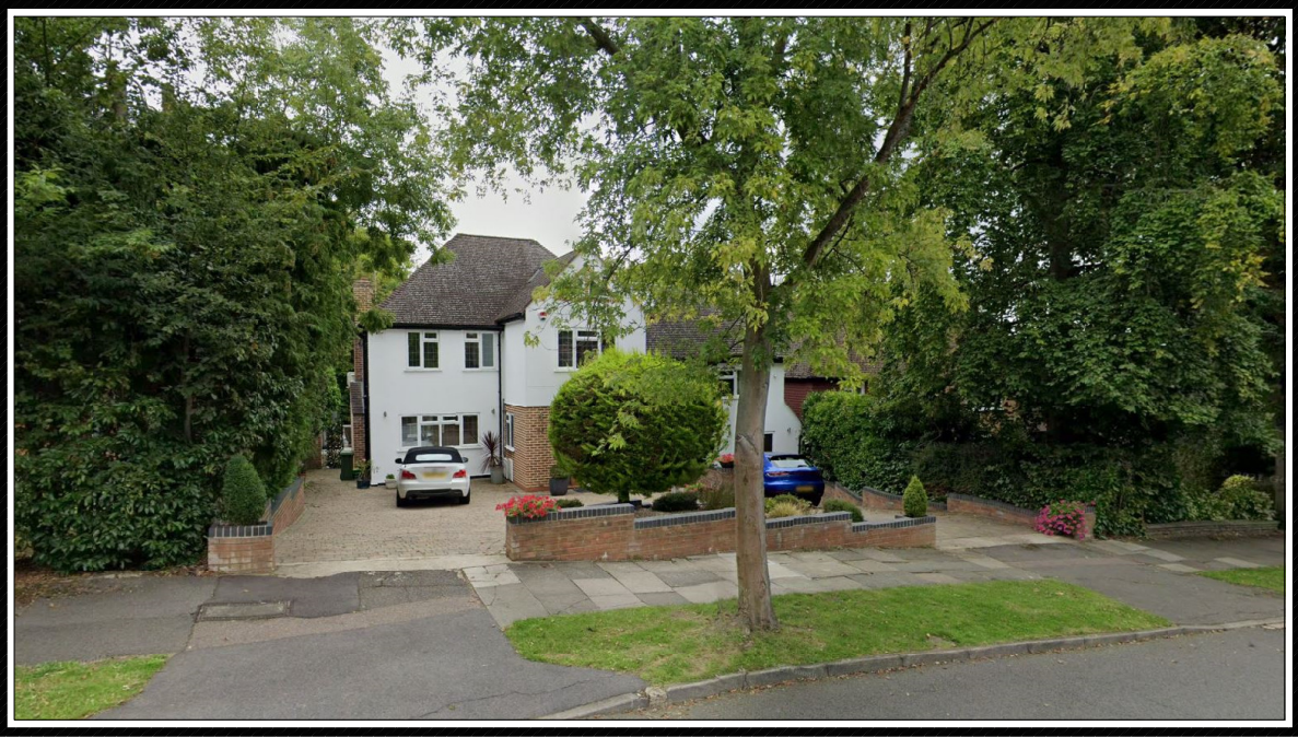
EXISTING STREET SCENE PHOTO
