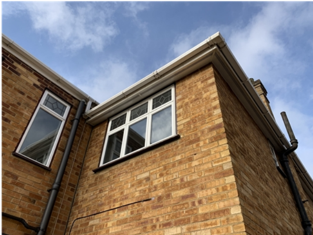
Views from rear patio looking towards drainage routes
