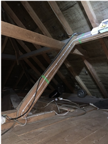
Views from existing loft
