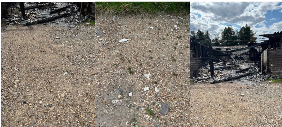
Photos - S2 showing fire damaged asbestos building and asbestos fragments littering the surface.
