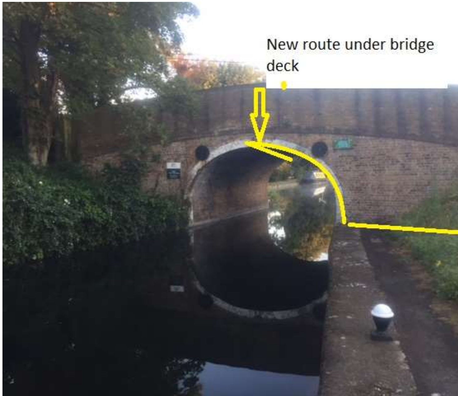
Photo 2 showing route of new duct installation to Iver Lane Bridge (Looking North).
