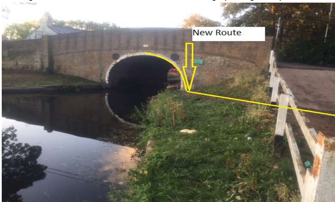
Photo 1 showing route of new duct installation to Iver Lane Bridge (looking South)
