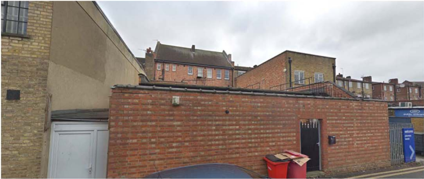
V2 - Rear Elevation of 173-175 Field End Road and Adjacent Buildings
