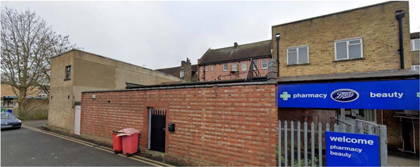
V3 - Rear Elevation of 173-175 Field End Road and Adjacent Buildings
