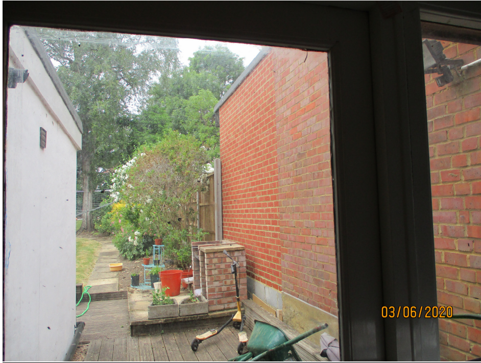
Image No.4: From inside the Laundry Room showing the two separate extensions (in two slightly different bricks) built on the rear of the neighbouring house.
