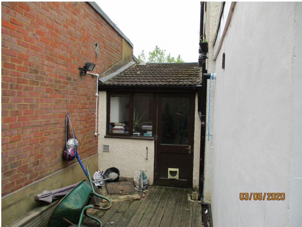
Image No.5: We propose converting this space into the new Kitchen.
