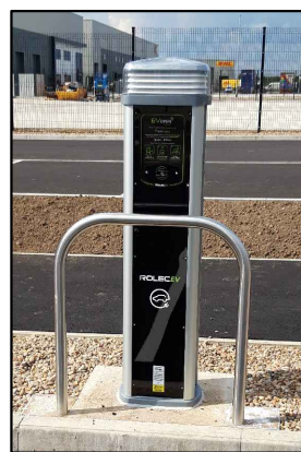
EV Charging Post with Bollard Protection Location: EV Charging spaces Note: Extent and type of protection to be confirmed by contractor. Refer to specification for EV post details.
