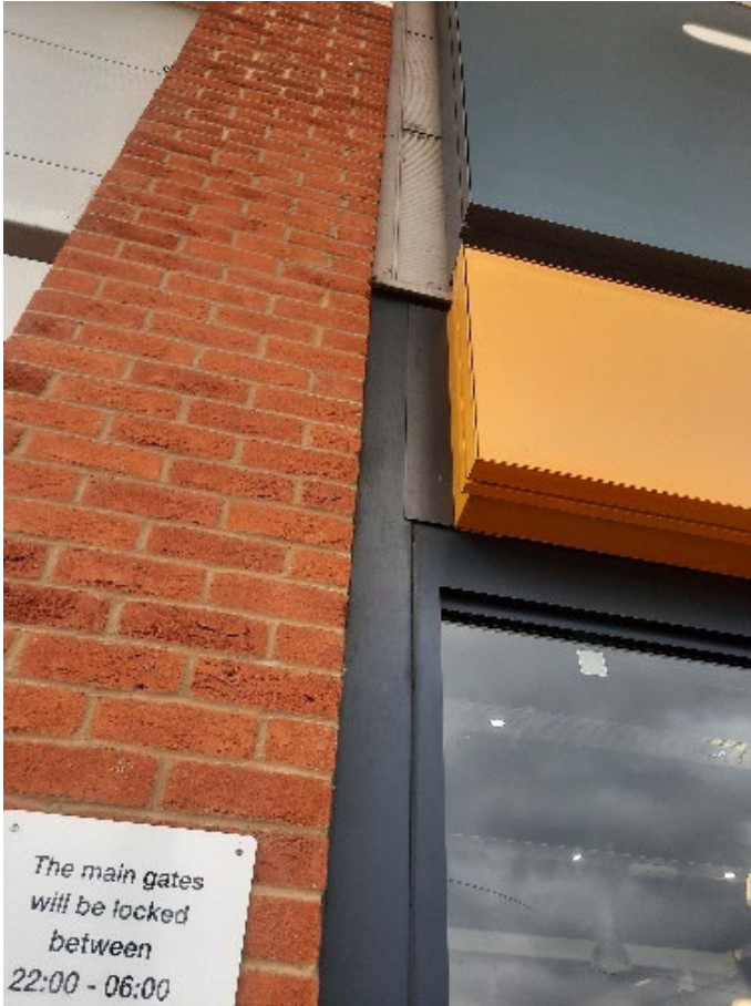
Photograph 8 (below): Gaps under and around metal cladding on the front and corners of all commercial units.
