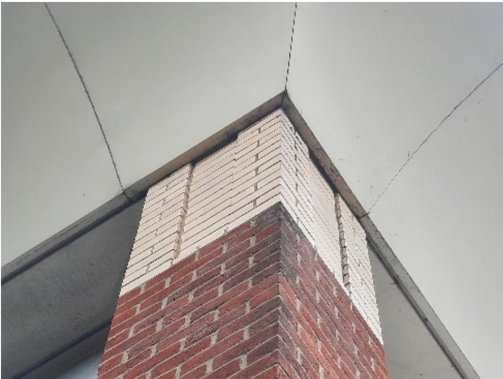
Photograph 8 (below): Gaps under and around metal cladding on the front and corners of all commercial units.
