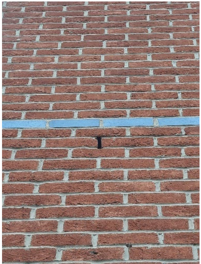
Photograph 6 (right): Weep hole in brickwork on the north elevation.
