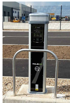
EV Charging Post with Bollard Protection Location: EV Charging spaces Extent and type of protection to be confirmed by contractor. Refer to specification for EV post details.
