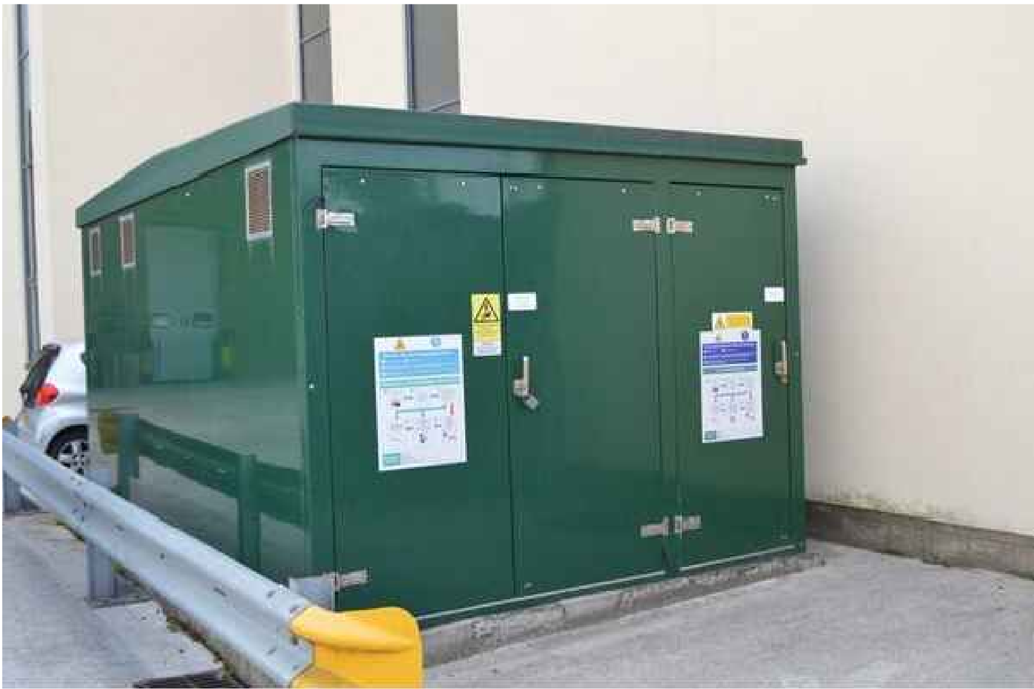
Extract A: Typical glass reinforced plastic housed substation to meet energy and power distributor's specification. Size: 4.0m x 4.0m x 3.0m high, with double-door aperture of 2.7m x 2.1m high. Colour: 18 B 25 (Merlin Grey or Green) to meet standard approved colours defined by energy and power distributor in accordance with BS 4800: 2011.
