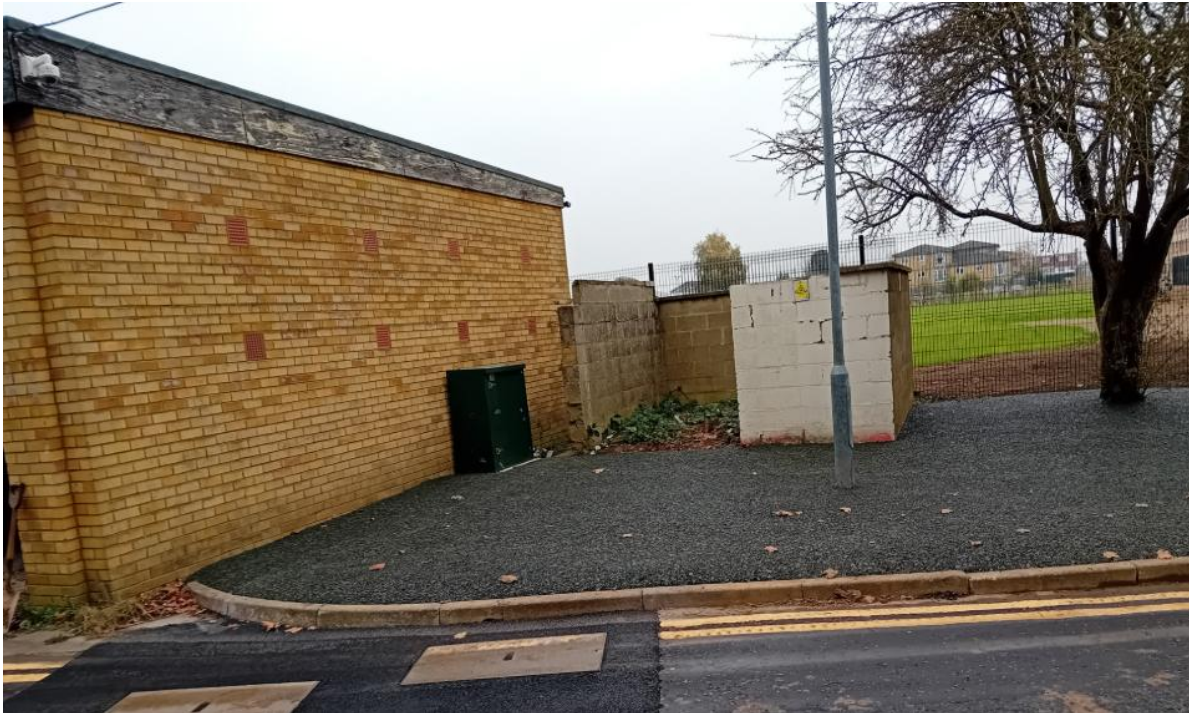
Figure 5 photo of location of WS 102 capped off with proprietary bonded granular rubber mulch
