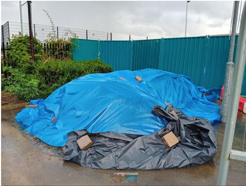
Figure 7 – photo of spoil heap / arisings from remediated area of WS 103
