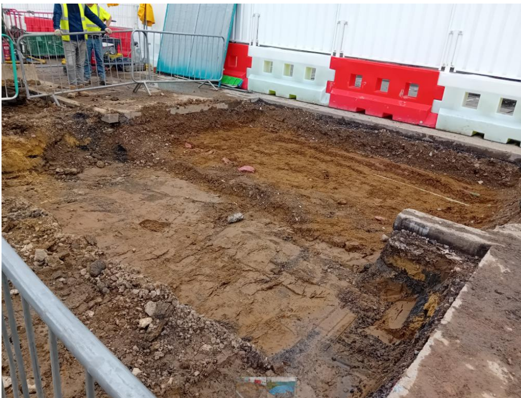
Figure 6 – photo of excavated remedial area of WS 103
