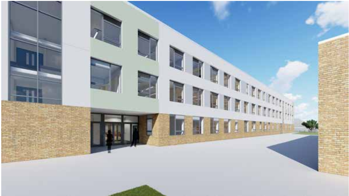
External Appearance - Main Student Entrance Approach (South Elevation)
