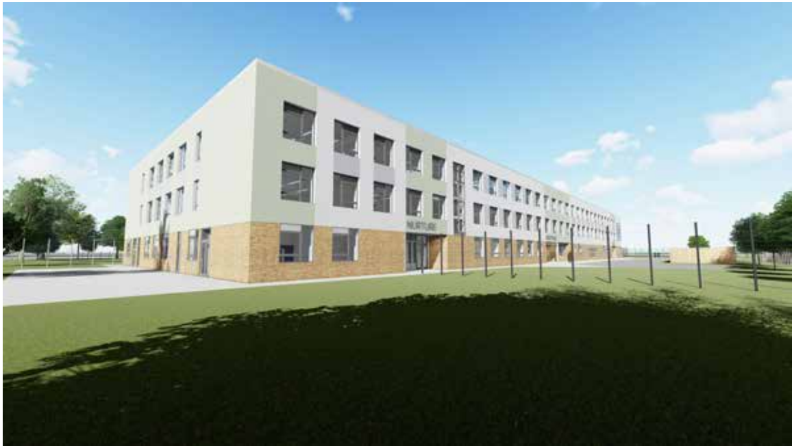
External Appearance - SEN Outdoor Provision (North East Corner)
