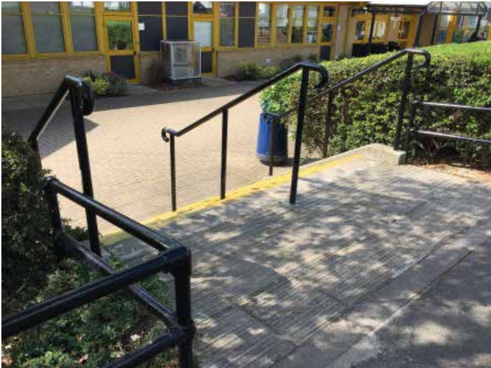
Steps from Pinkwell Lane to Main Site
