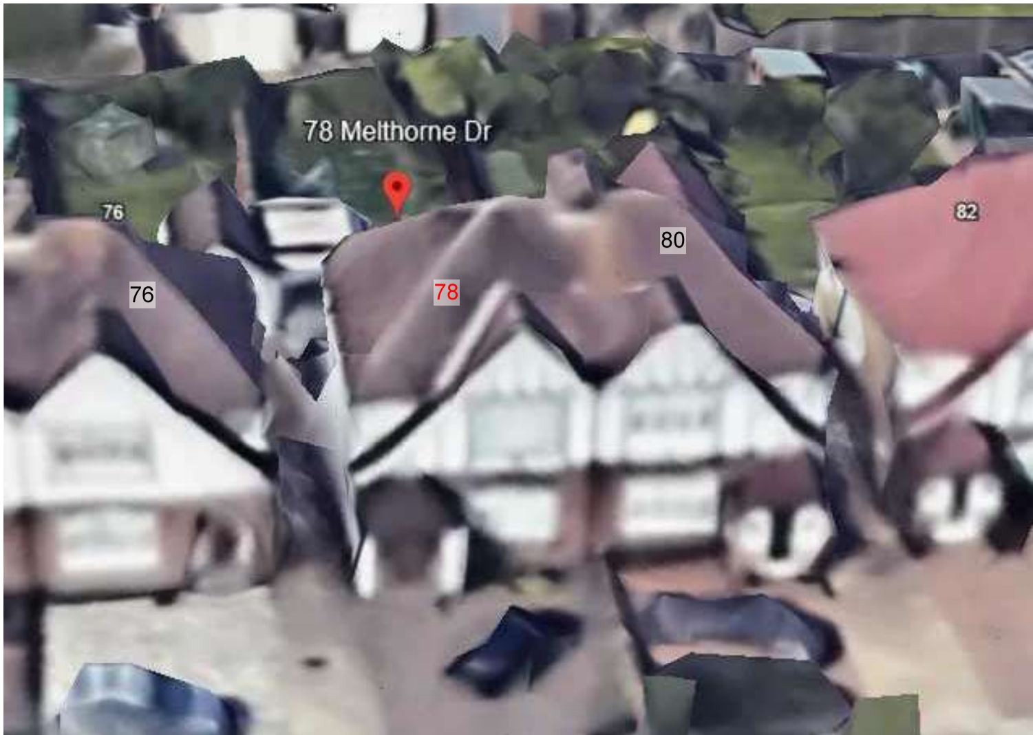
Front aerial view
