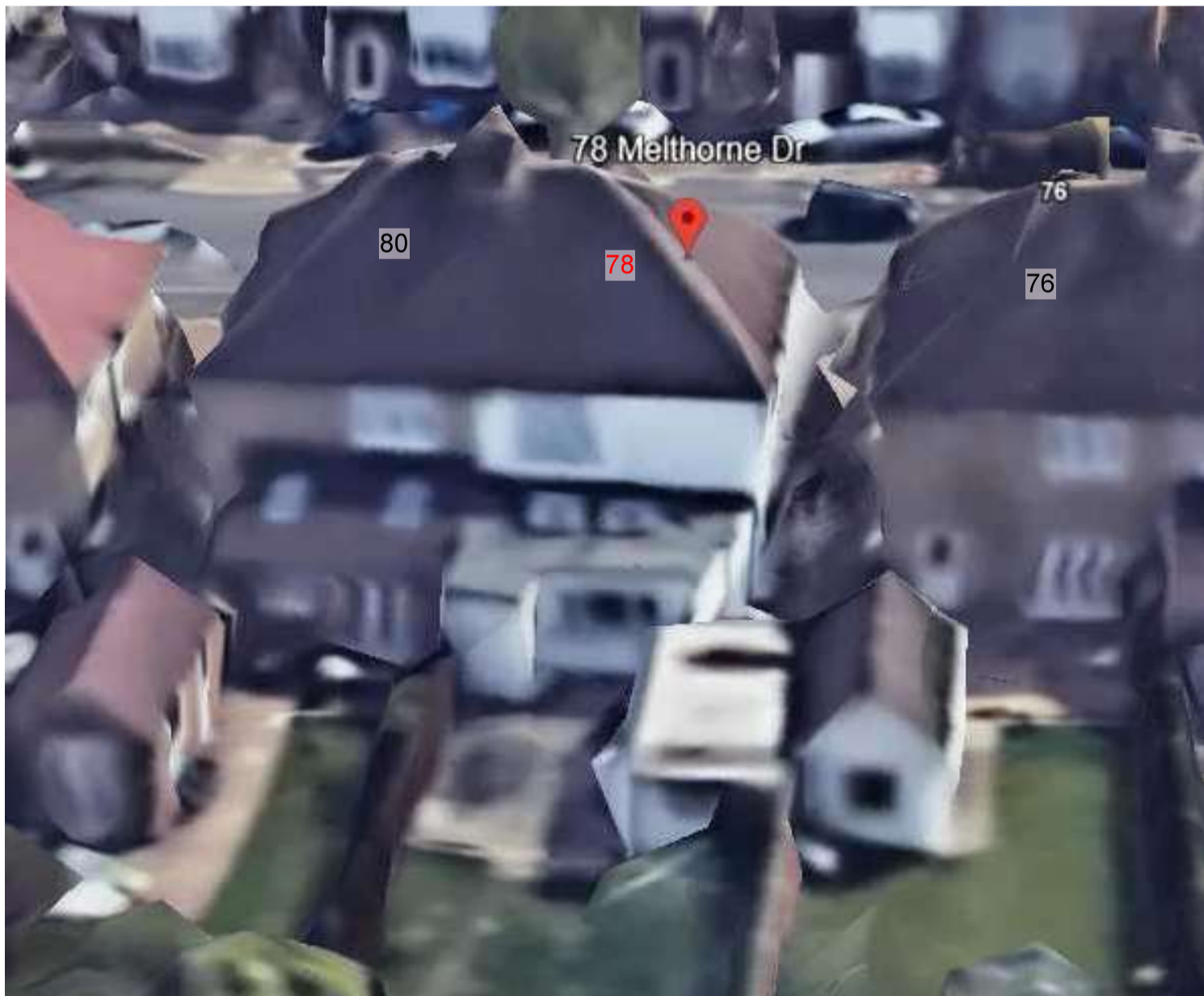
Rear aerial view
