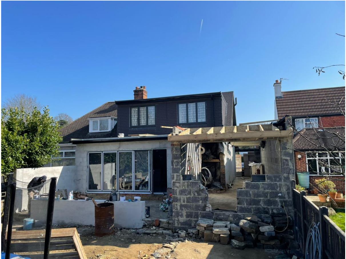
Figure 3 - view from rear (currently building)
