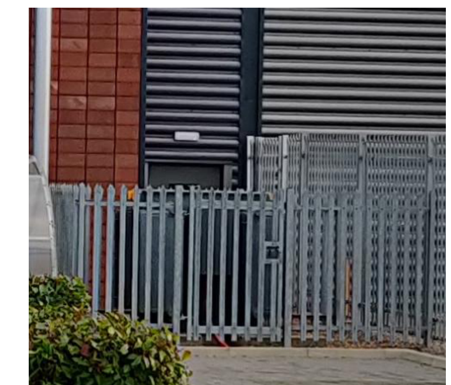
Above image: 1.8m Existing Palisade Fencing
