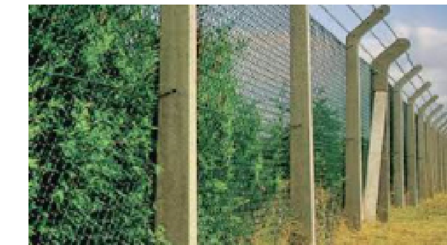
Above image: 2m Existing Chain Link Fence with Concrete Posts
