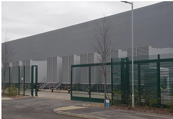
IMAGE ABOVE: SHOWING EXAMPLE OF EXTERNAL GENERATORS
