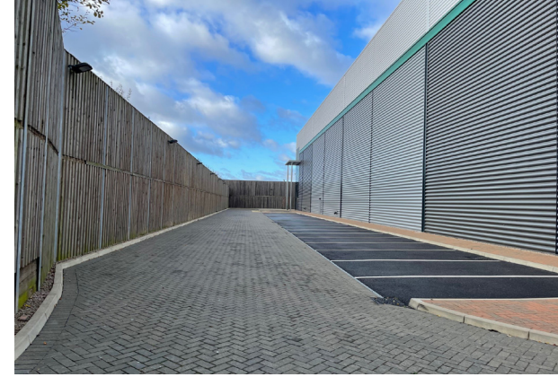
IMAGE ABOVE: SHOWINGEXAMPLE OF ACOUSTIC FENCE
