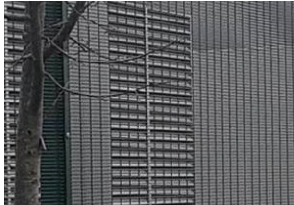
IMAGE ABOVE: SHOWING EXAMPLE OF EXTERNAL SECURITY FENCE
