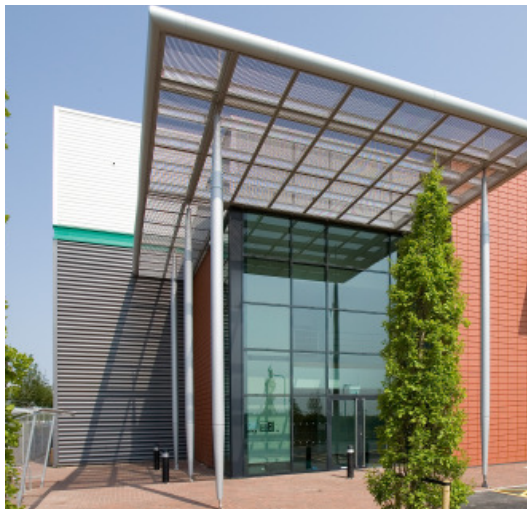
Metal Cladding, Curtain Walling, Terracotta Cladding
