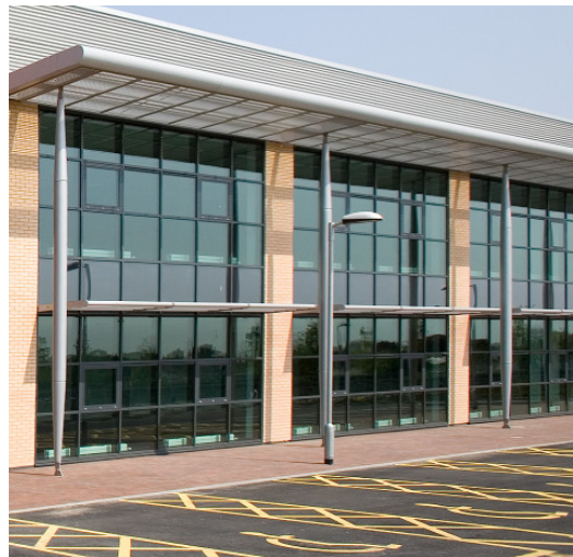
Metal Cladding, Curtain Walling, Brickwork Piers
