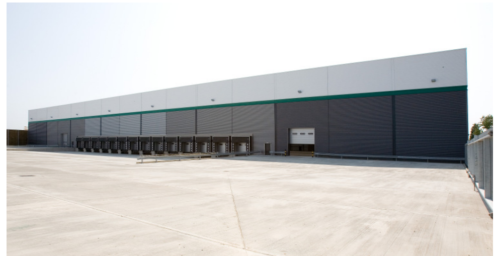
Metal Cladding, Loading Doors
